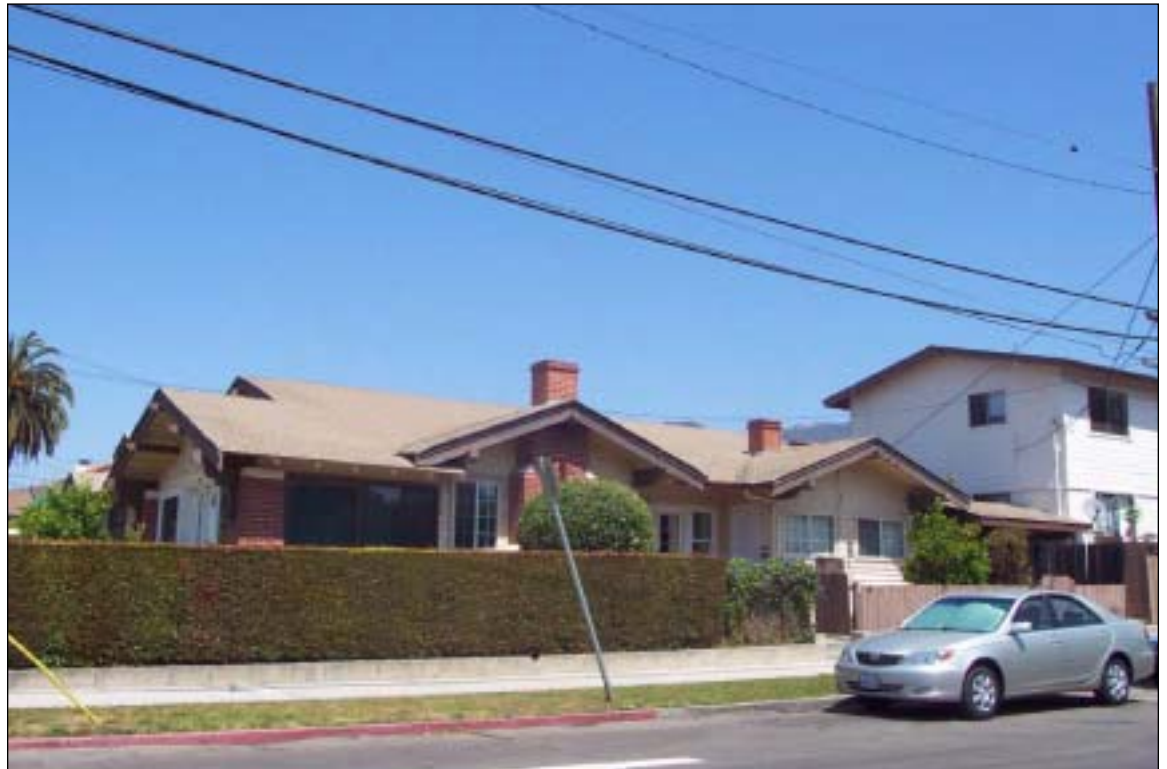
7 unit building on far right
